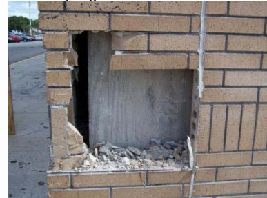
Plant City High School
